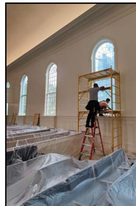
Last of the old windows being removed
